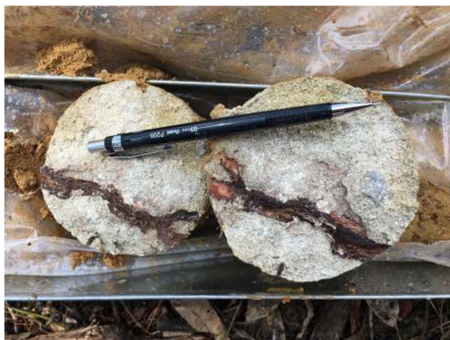
Fig. 13 Large tree roots recorded penetrating along bedding planes in sandstone at 4.5 mbgl in GB20a
