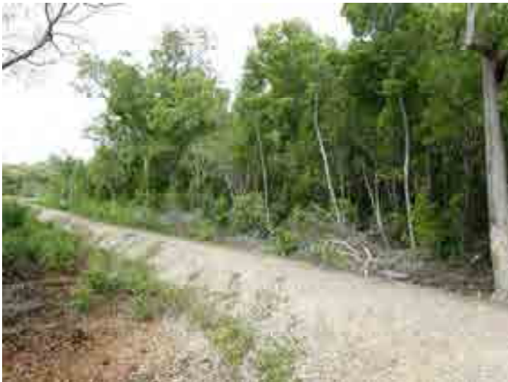
Photograph 188. Bunding on Boigu Island for the purpose of land reclamation.
